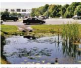
Orchard pond with gentle side slopes provides a safe feature with easy access for maintenance, Florida, USA
