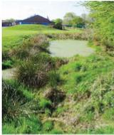
Algae in a SuDS pond is common in the first year or two after construction. (Photocourtesy)
